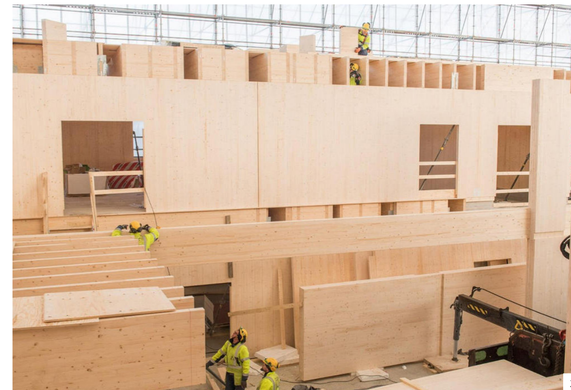
1. PV panelen 2. Cross Laminated Timber bouwsysteem
